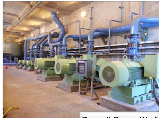
Pump & Piping Work
